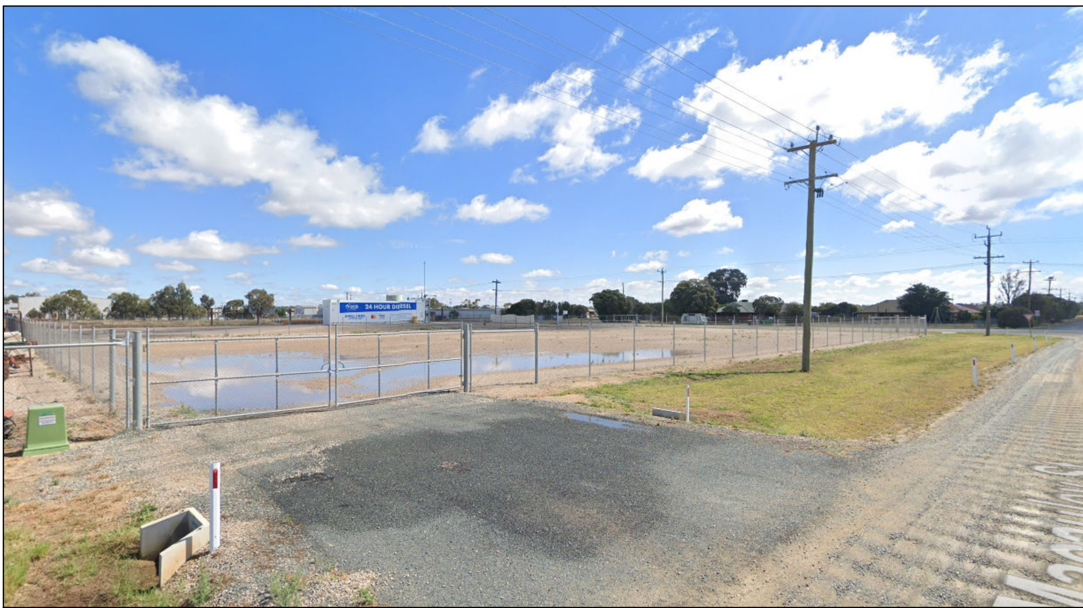
SITE VIEW B - LOOKING NORTH
