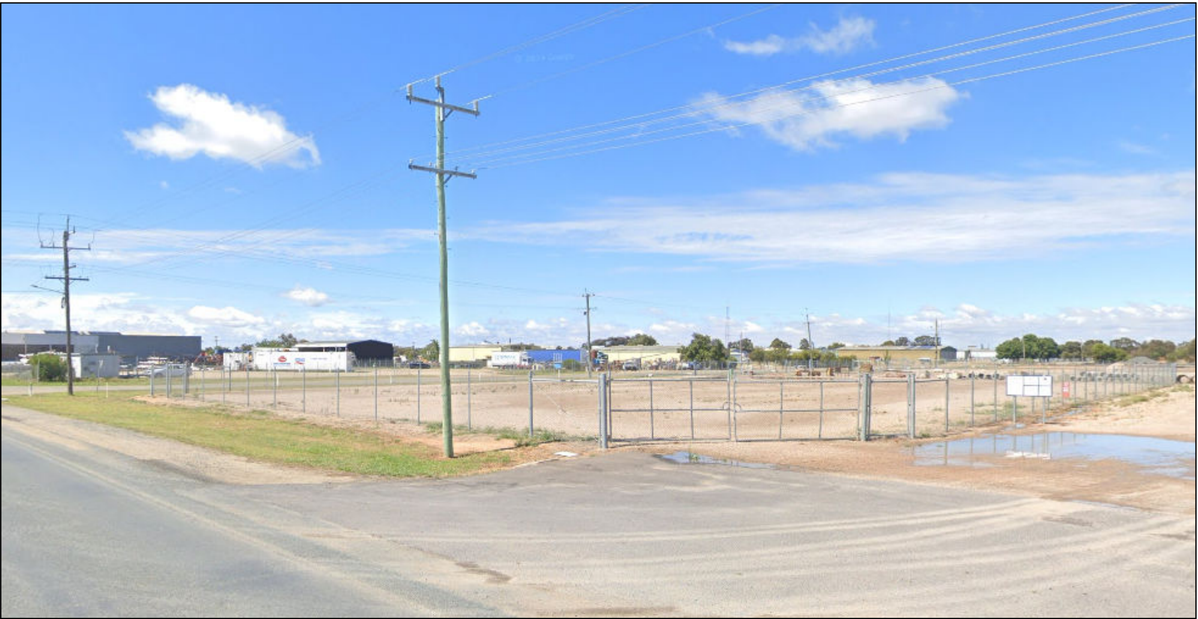
SITE VIEW A LOOKING SOUTH
